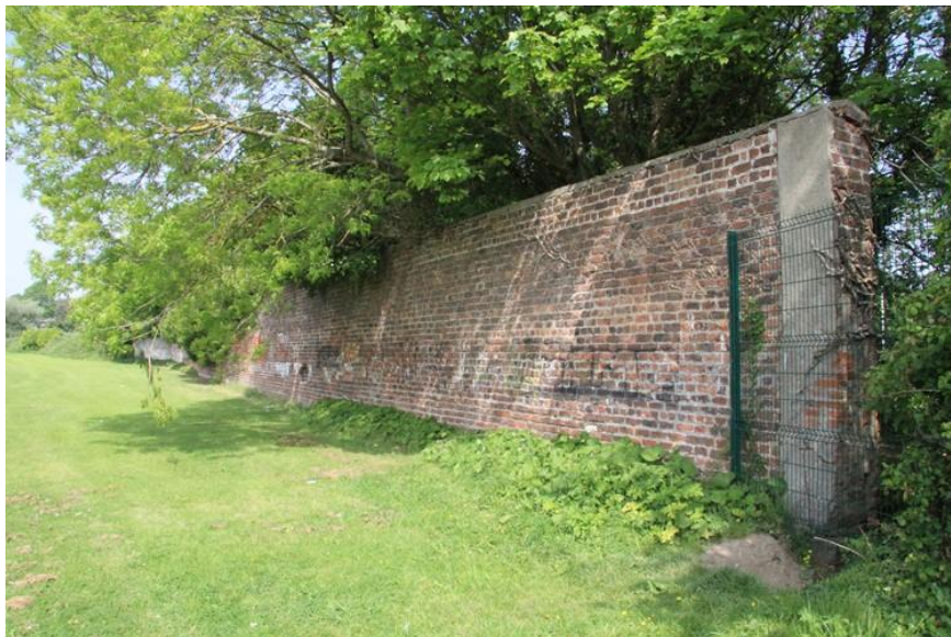
Plate 10: Brick-faced wall near northern boundary
