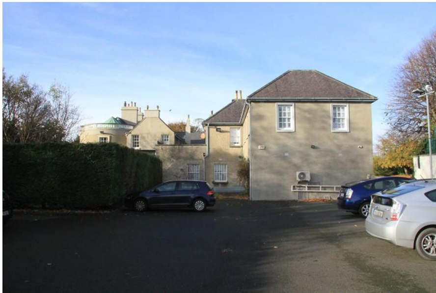
Plate 7: Eastern elevation of Sybil Hill House
