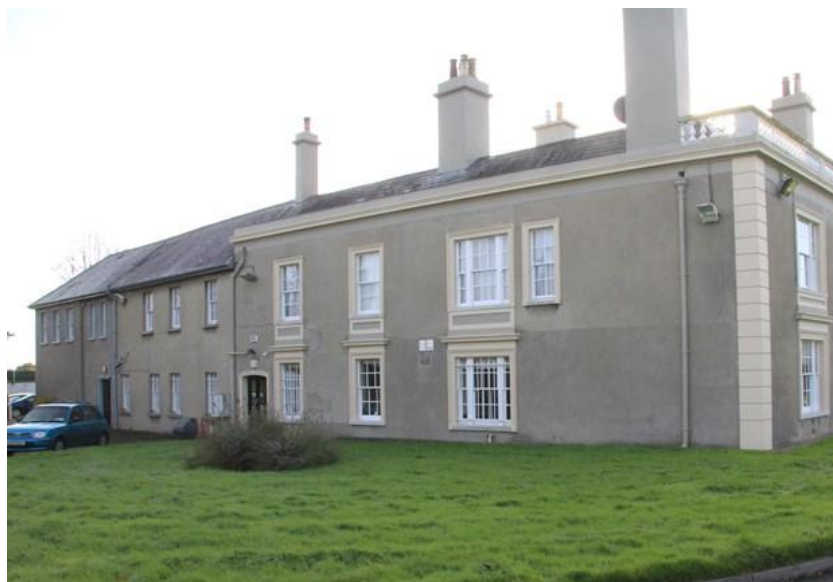
Plate 6: Northern elevation of Sybil Hill House
